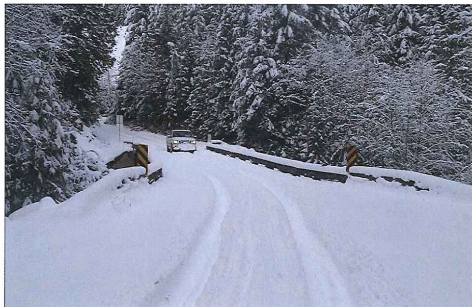
CK2445 Approach Left Bank
