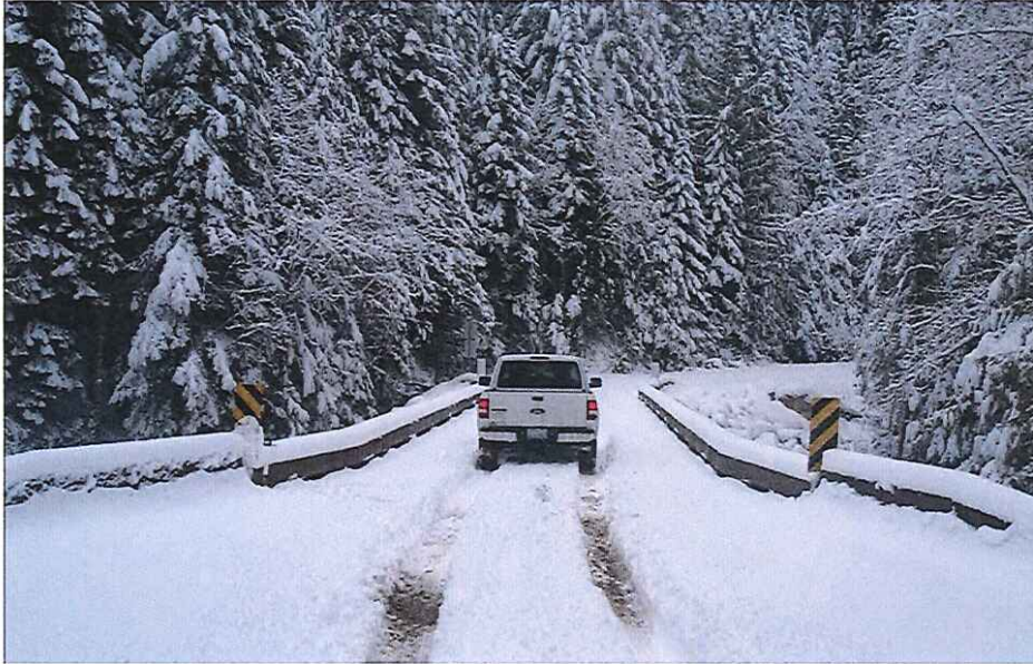
CK2445 Approach Right Bank
