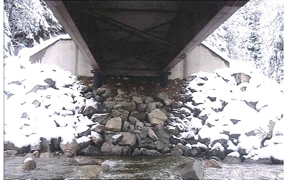
CK2445 Abutment Left Bank
