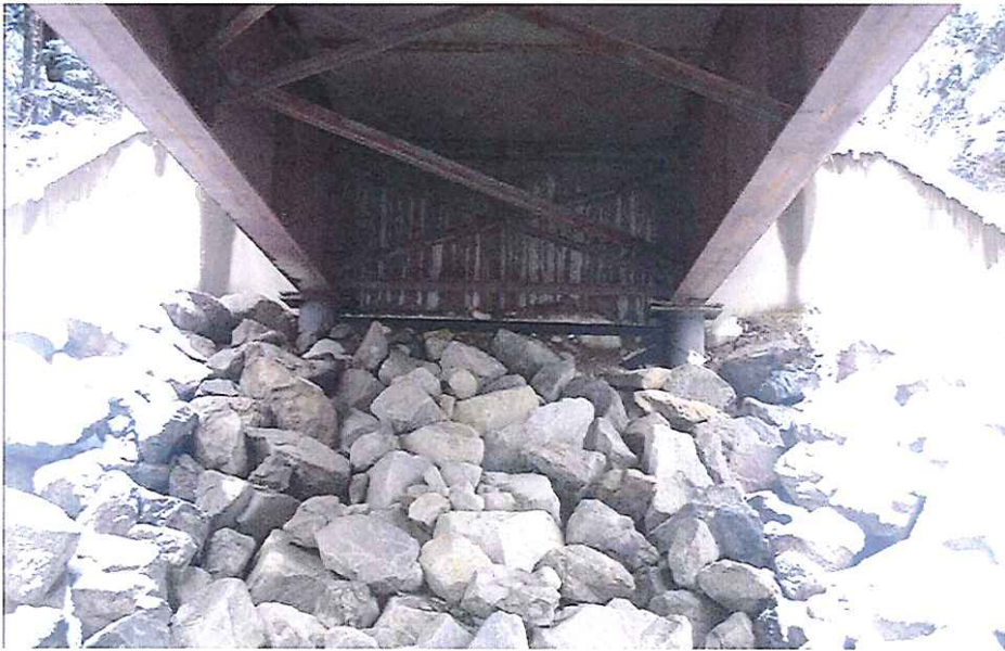
CK2445 Abutment Righth Bank
