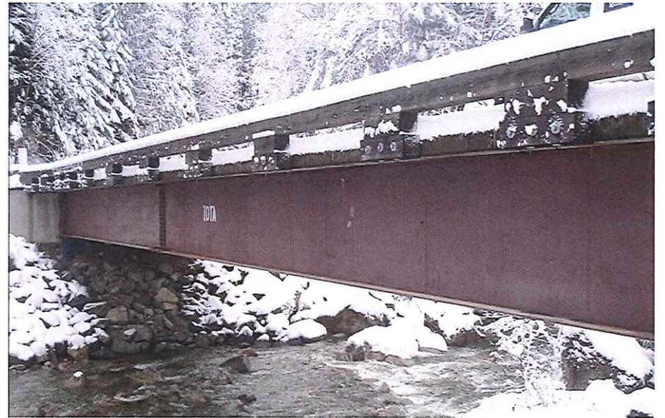
CK2445 Crossing Upstream
